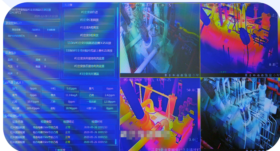
Execution of inspection tasks
