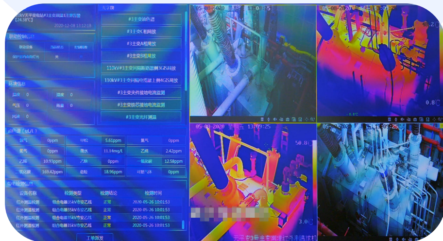
Execution of inspection tasks
