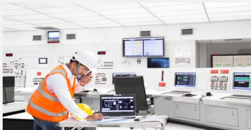
Heavy workload of operation and maintenance, insufficient carrying capacity of operation and inspection work
